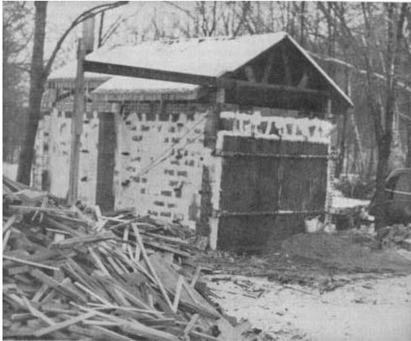
**Figure 41.** Experimental single wall, masonry kiln (Toole et al., 1961).
