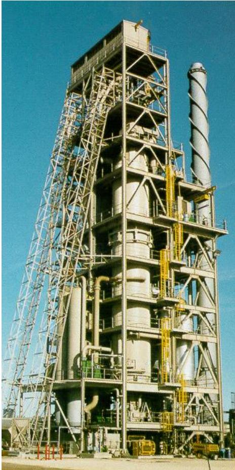
**Figure 57.** Lurgi process - charcoal production plant in Bunbury, Western Australia (<http://www.biochar.bioenergylists.org/files/Gronli.pdf>, date accessed: Nov. 13, 2010).
