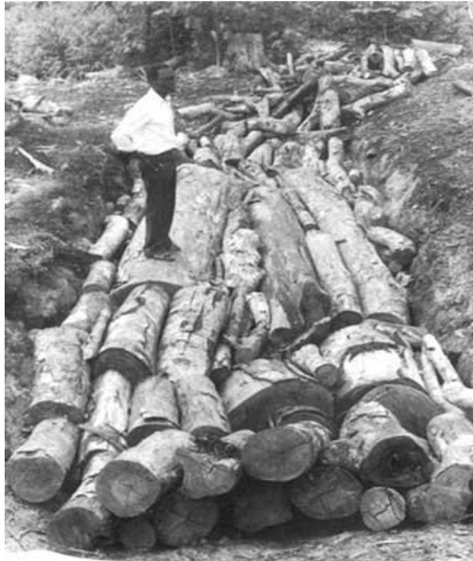
**Figure 36.** Biochar pit showing logs placed lengthwise across the crib (FAO, 1987). *Image courtesy of the Food and Agriculture Organization of the United Nations.*
