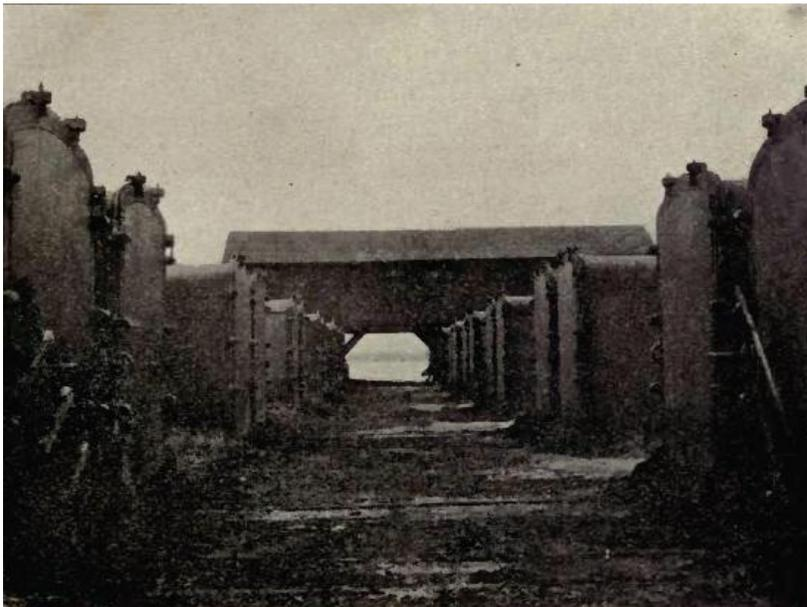
**Figure 52.** Looking down an alley between two sets of cooling ovens, Cadillac MI (Brown 1917).
