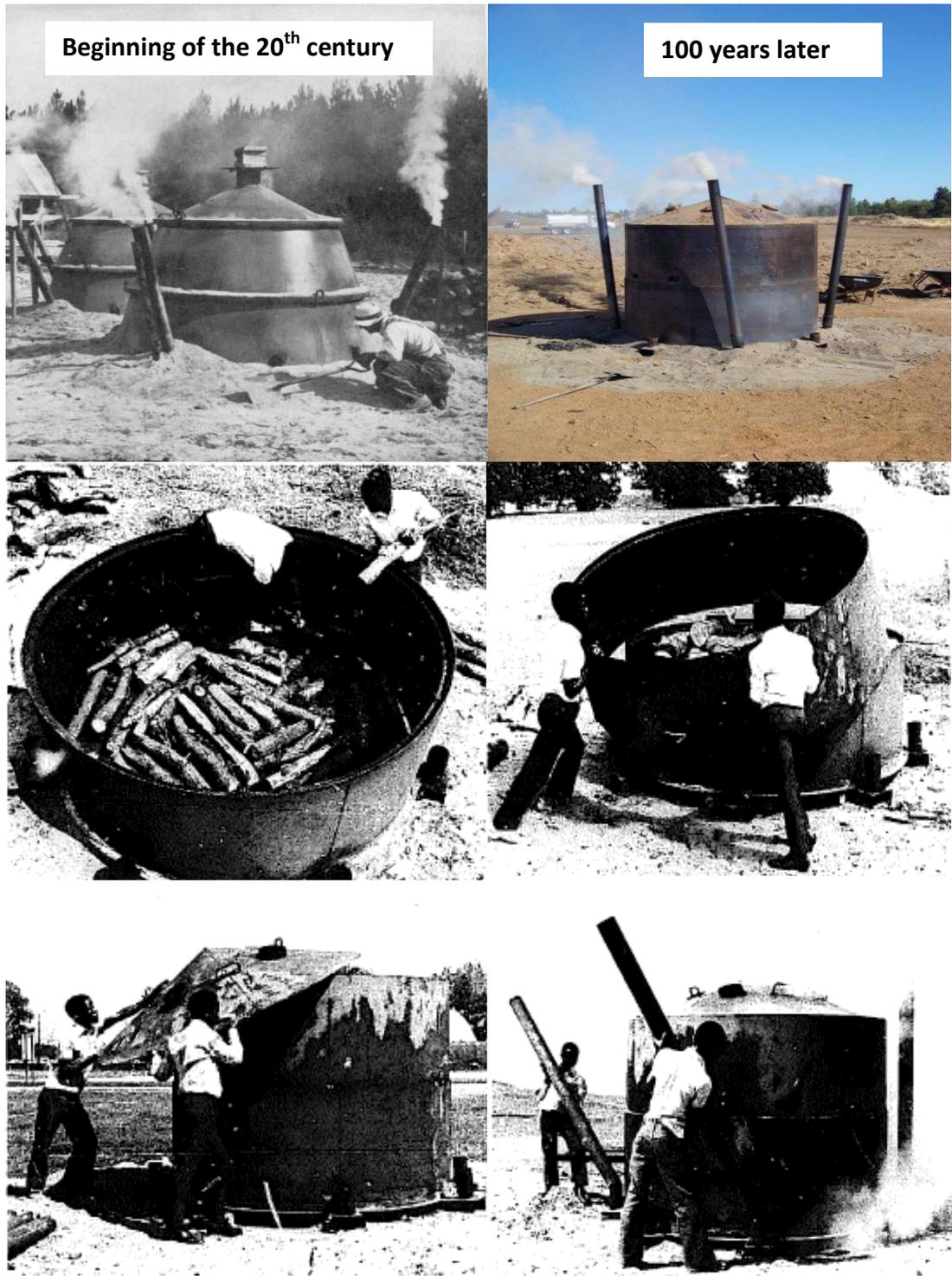
**Figure 24.** Examples of portable metal kilns (kilns assembled from portable sections) (Paddon and Harker, 1980).
