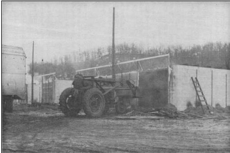
**Figure 28.** Tractor with a scoop being used to discharge a kiln (Toole et al., 1961).
